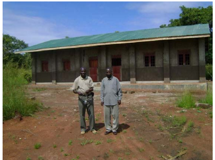
Bishop Francis (right) with our Project Manager Dan Kure standing in front of the newly completed school in Rokon
